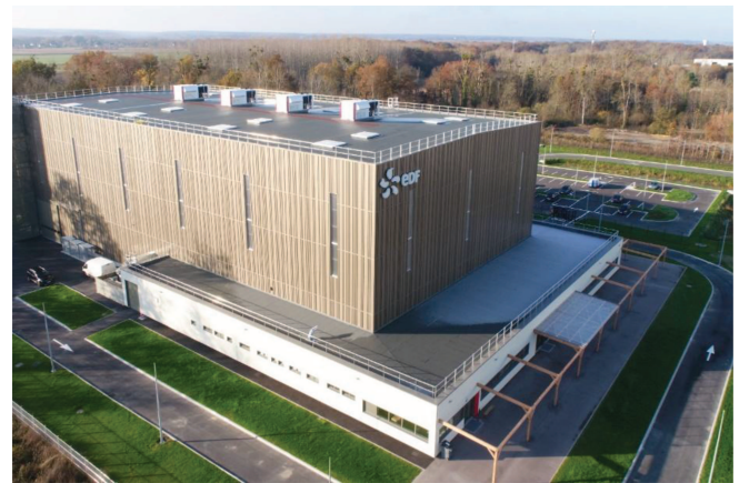
Fig. 3. EDF's industrial demonstrator.
