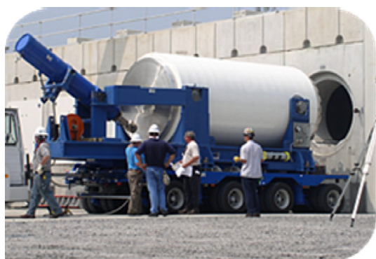
Fig. 5. Loading a canister into a horizontal concrete storage module (Courtesy of Areva TN Inc).
