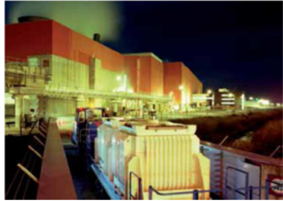
Fig. 1. Centralised storage pond (Courtesy of Sellafield Ltd).
